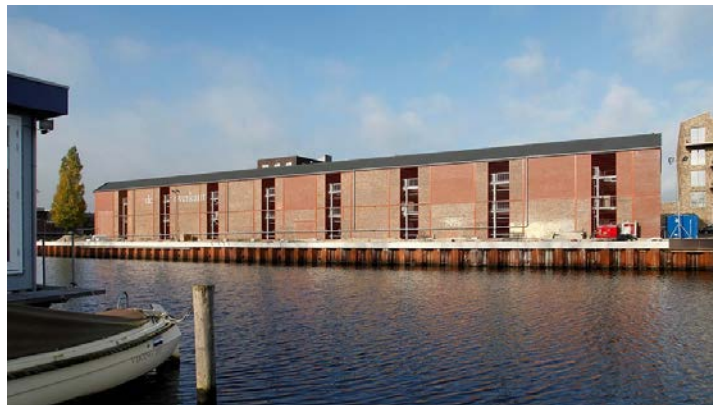
Parkeergarage in monumentale loods
